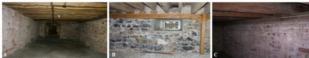
Figure 3. Masonry walls and timber slab system in the Beylerbeyi Palace ((A and B) foundation floor; (C) second floor).
