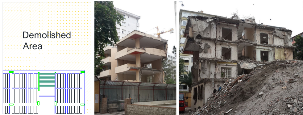
FIGURE 15 The studied building after the fourth ground demolishing
