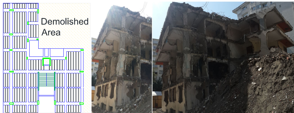
FIGURE 11 The studied building after the second ground demolishing
