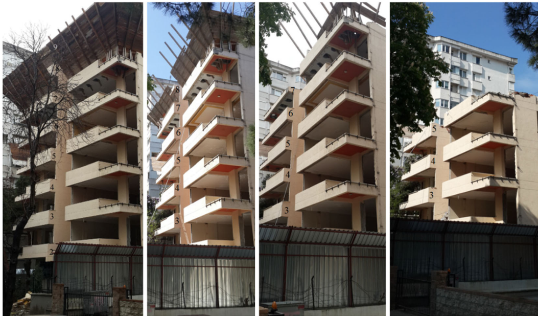
FIGURE 5 Floor removal in the studied building
