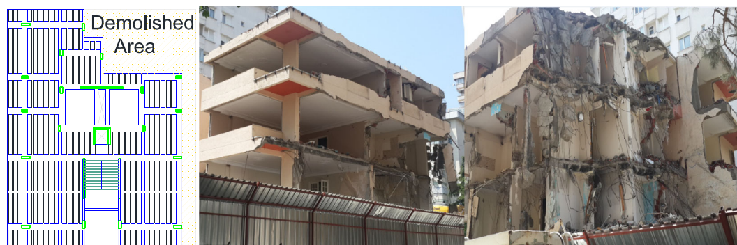
FIGURE 9 The studied building after the first ground demolishing
