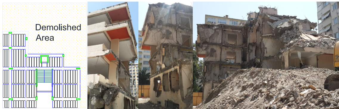
FIGURE 13 The studied building after the third ground demolishing
